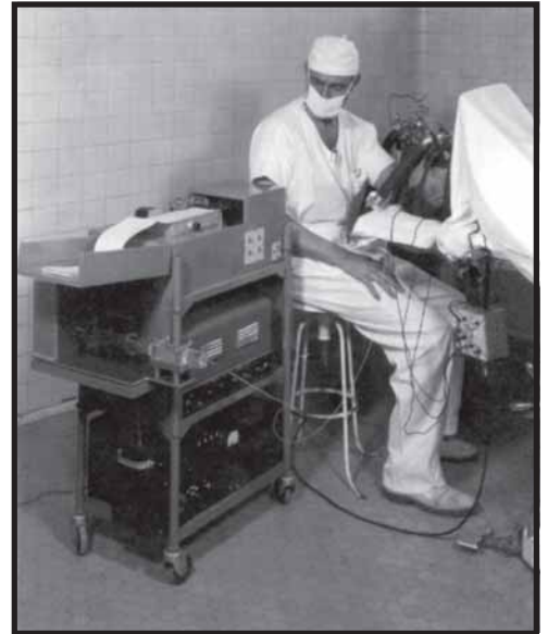
Fig. 3: Donald Sotero, a colleague of Albert Faulconer, with the servo-controlled anesthesia machine. This model automatically delivered pentothal anesthesia. The syringe pump is on the left side of the servo-anesthesia machine. This system was also adopted for administration of ether anesthesia, wherein ether was injected from the syringe pump into the inspiratory limb of the anesthesia circuit. (From Rehder K, Southorn P, Sessler A: Art to Science. Mayo Foundation for Medical Education and Research, Rochester, Minnesota, 2000. By permission of Mayo Foundation for Medical Education and Research).
